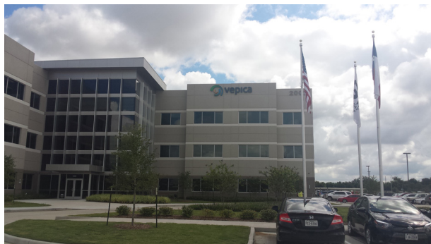
Figure 3. Design information from three offices was synchronised into a central database server to create the 3D model.
