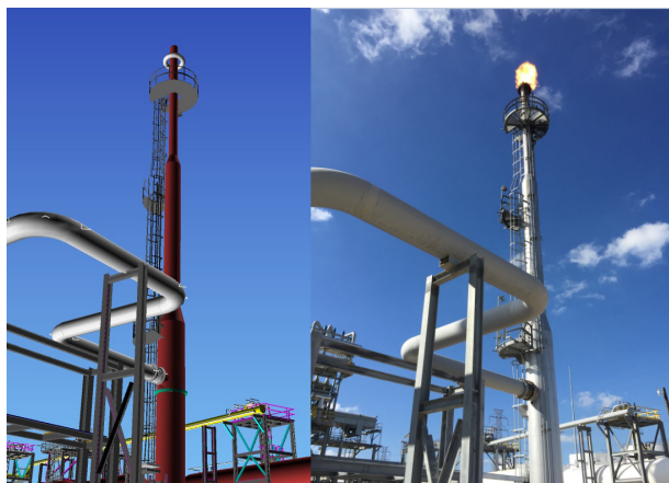
Figure 4. The client used CADWorx's 3D model for reviews during the fabrication phase of the project.
