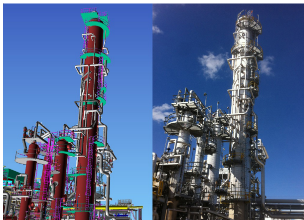
Figure 5. The 3D visualisation matches the actual as-built facility.
